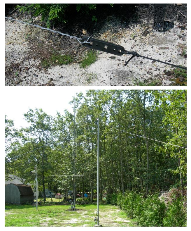
The 80 and 60 meter radials do not run at 90 degree angles to one another because of space limitations. Instead they are only a few feet apart at their ground anchors. Underground PVC conduit carries the RG8 feedline to a central connection point, where a remote conduit switch can select a GAP Titan vertical antenna or the dual band NVIS.
