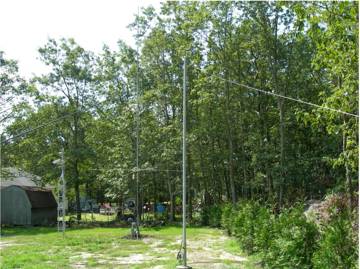
The 80 and 60 meter radials do not run at 90 degree angles to one another because of space limitations. Instead they are only a few feet apart at their ground anchors.
